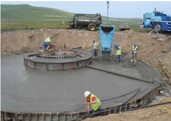
Above: the huge base is formed to hold the turbine tower. Below: the installation nearing completion.
