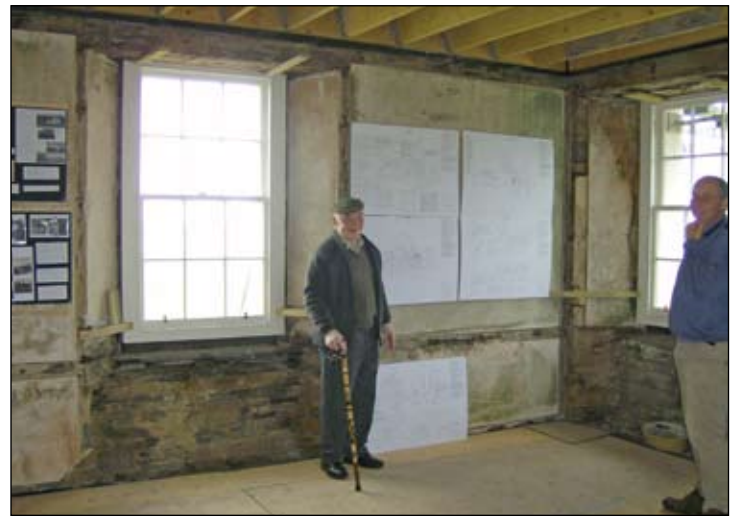
Plans for the completed house were displayed on the walls, as were old photographs of people at Brough. Pictured chatting are Jeemie Fergus and Douglas Leslie.
